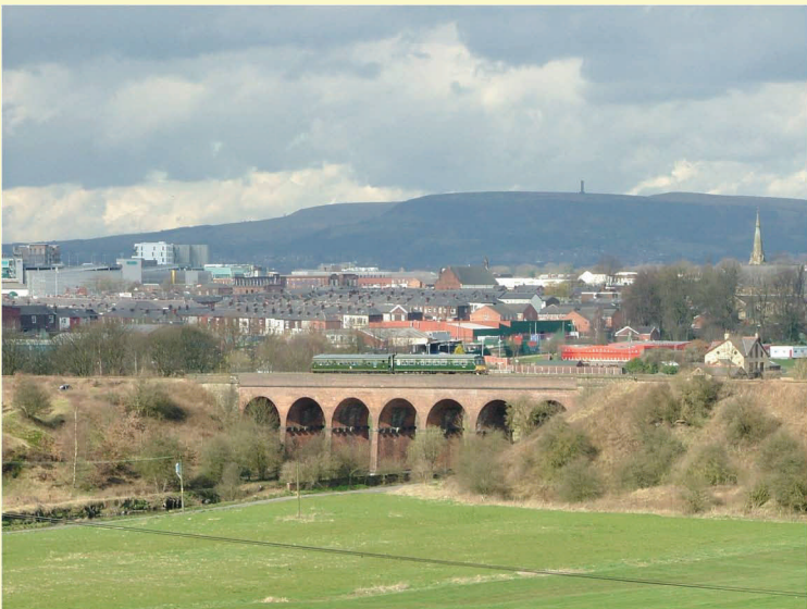
The 101 set crossing Heap Bridge Viaduct
